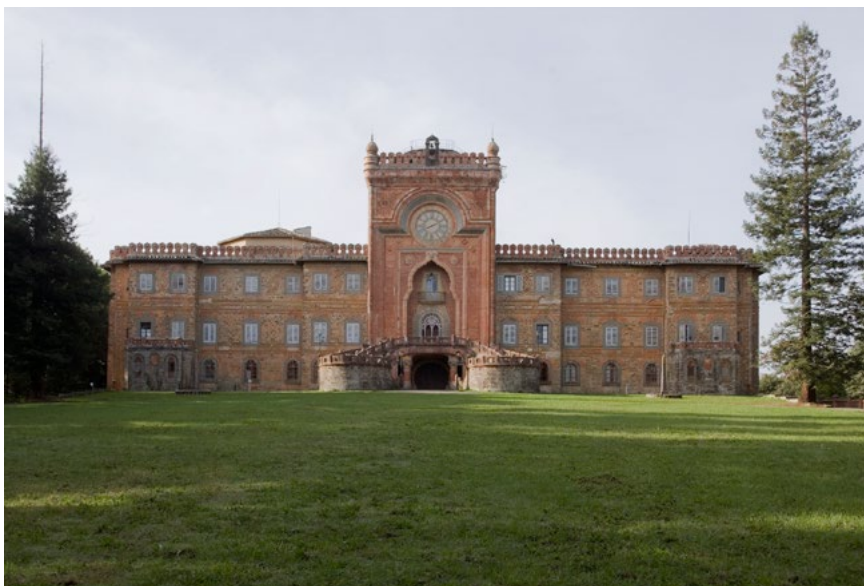
Figure 1 Regello, Villa of Sammezzano, exterior view (Ferdinando Panciatichi Ximenes d'Aragone, 1840s-1910s). © Bildarchiv Foto Marburg / Rabatti & Domingie Photography.
